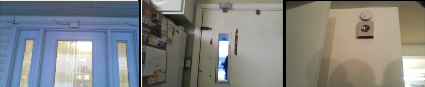
INTRUSION STATION OVER OUTSIDE DOOR DOOR STATION AND ARM/SUSPENSION REMINDER SMOKE AND SPEAKER STATIONS
